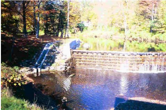
Green River Dam and Fishway
