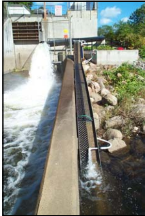
Kinneytown Hydro FERC # 6985 Naugatuck R. CT Akwadrain and Enkamat Substrate
