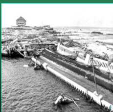
Suffolk County shoreline after the 1938 "Long Island Express" hurricane.
