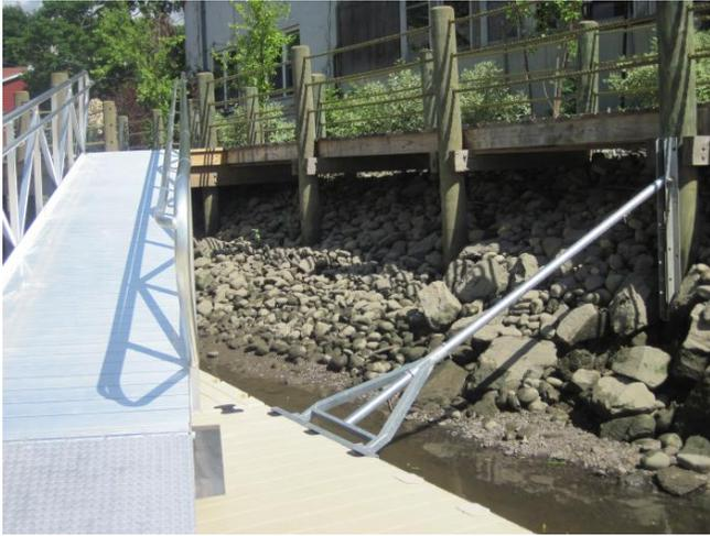
Figure 5: Ramp leading to floating dock allows access. The elevated walkway allows for a sloped shoreline and protective rip-rap to be maintained underneath.
