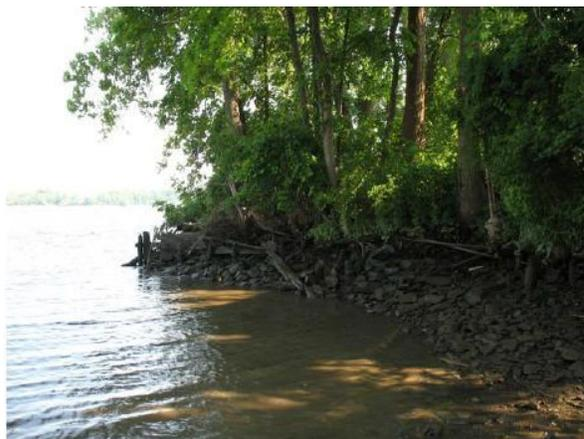
Figure 2: Shoreline was previously protected with rip-rap and degraded pilings on the southwest shore.
