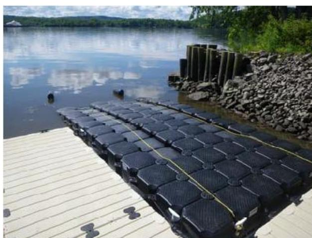
**Figure 4: Floating dock with shoreline rip rap and pilings visible in the background.**
