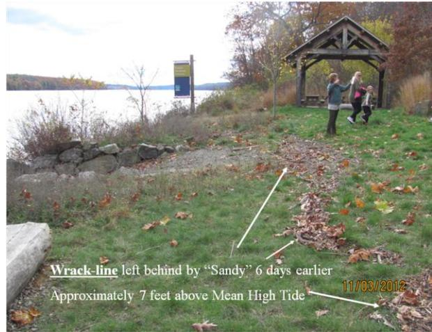
**Figure 6: Despite a wrack line 7 feet above the mean high tide, the shoreline survived Hurricane Sandy with no damage.**
