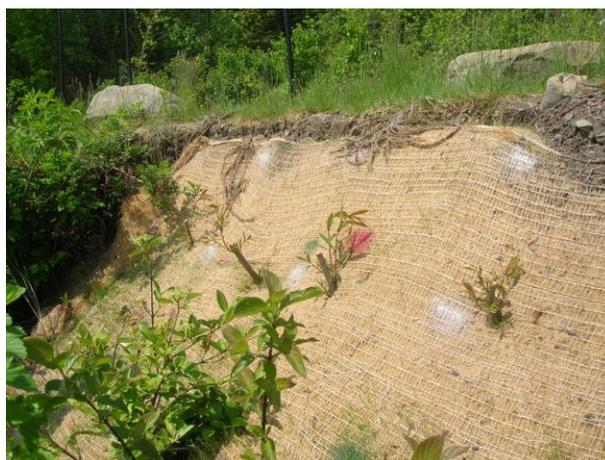
Figure 4: Live stakes and erosion control mats used to repair damage following a storm in April 2007.
