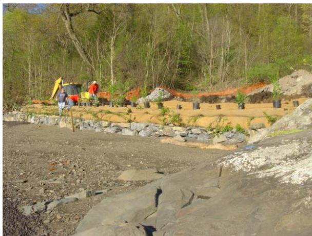
Figure 3: Soft gabions installed in May 2006.
