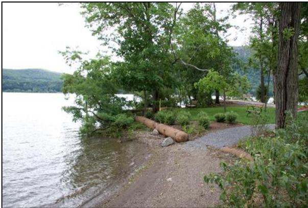
Figure 2: Newly constructed coir rolls at the edge of the shoreline.
