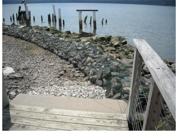
Figure 4: Additional rock added to the sill in 2007 to prevent erosion and control driftwood.
