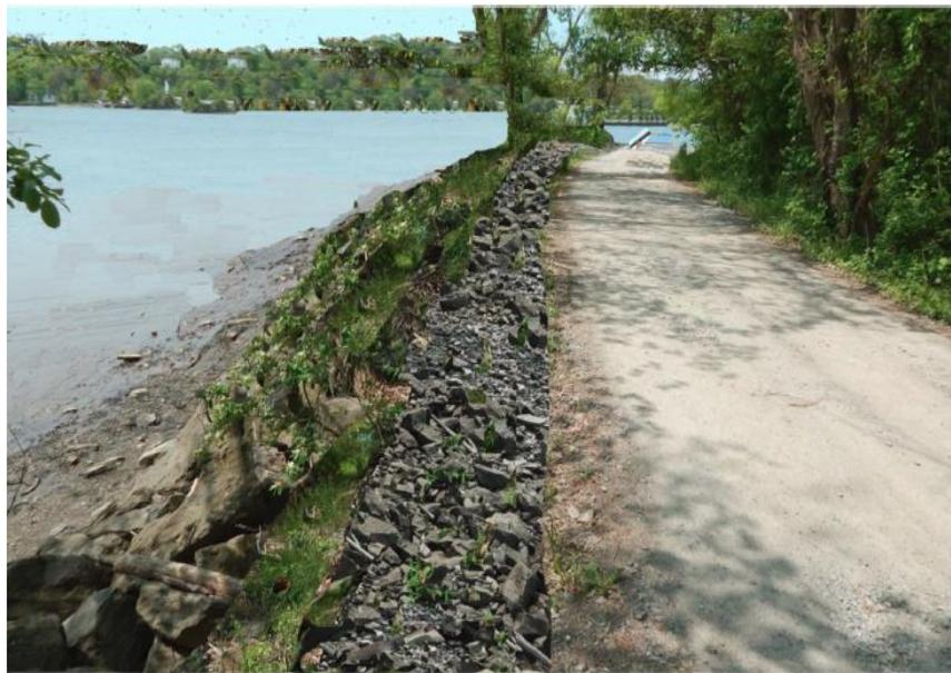
**Figure 3. Visualization, created by BlueShore Engineering, of existing stone bulkhead to left, native plantings by plug and wattles in middle, and rock armoring along southern shoreline sandwiched parallel to Ferry Road (looking west). Trees along the stacked stone wall will be replaced with low growing vegetation to prevent destabilization of the road when trees topple over.**
